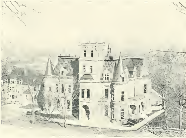
RESIDENCE OF MR. DUNCAN MCINTYRE.
